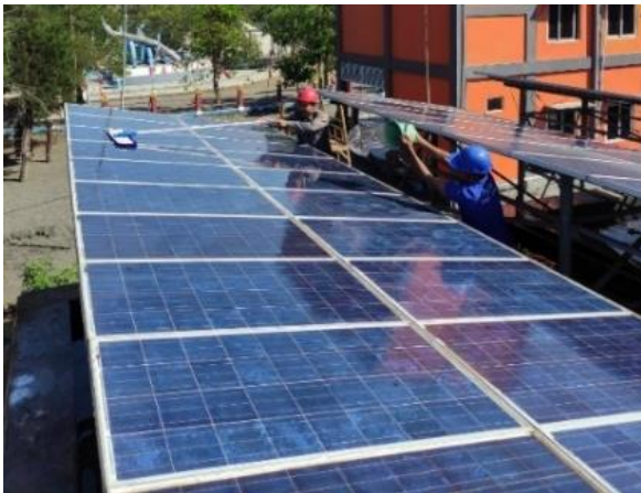
Fig.7. Solar Panel Maintenance
